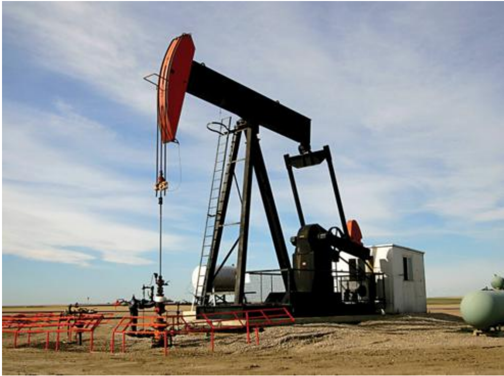
Figure 4.3: An oil-rig constructed at a well location.
