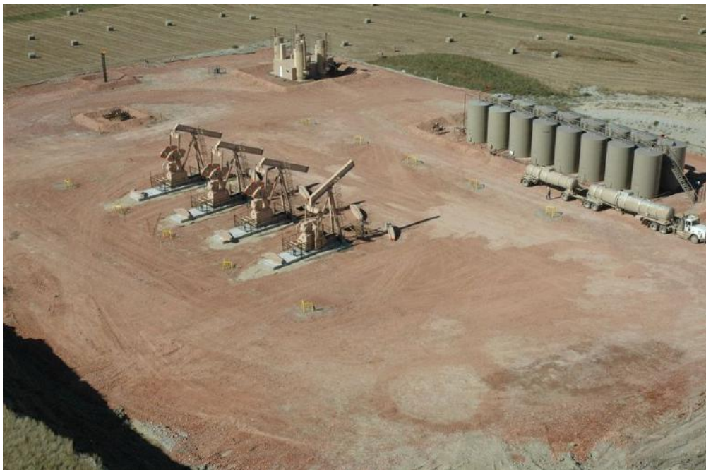
Figure 4.4: A multi-well pad site containing four wells.
